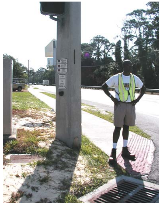
Push button is located away from the walkway
